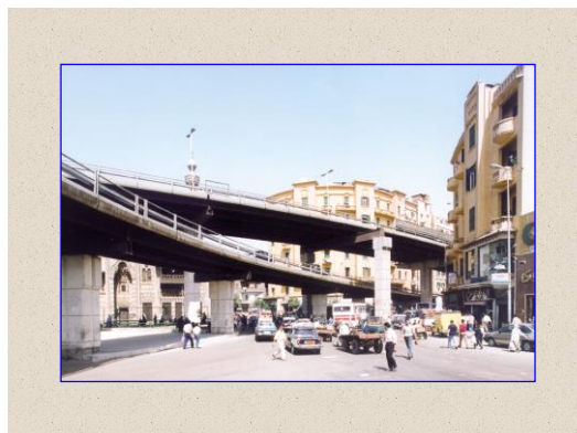
Figure 2: Bad sight seeing of El Azhar steel bridge
